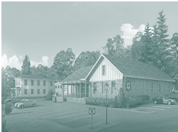
The new Willistown Township Police Department building is currently under construction.
